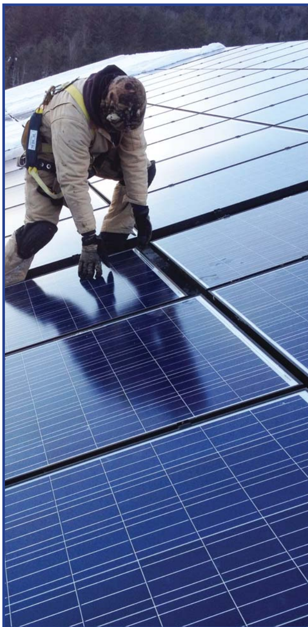
Photo: Aegis Renewable Energy
