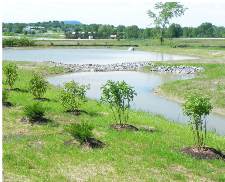
Right: Constructed gravel wetland in Ferrisburgh.
