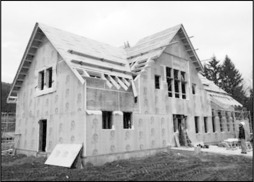
New Town Office under construction, Dec. 2015.
