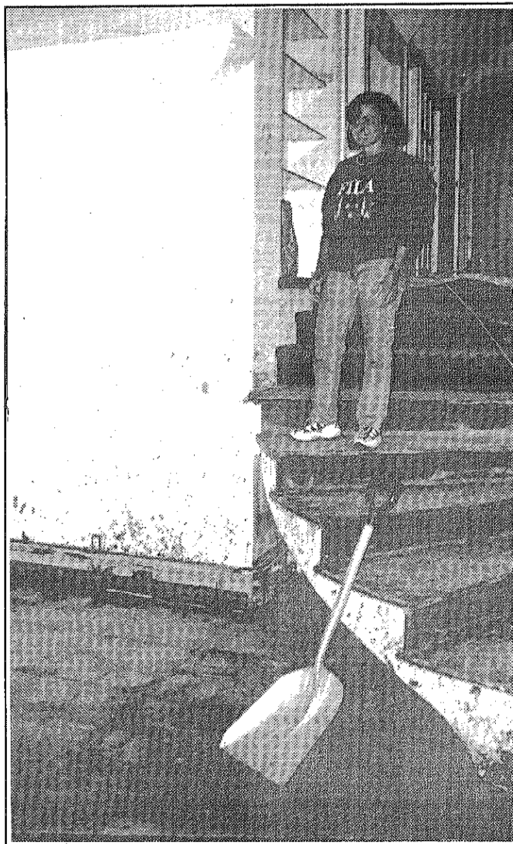
Marta Marble, Waitsfield, at the top of the steps to her living room. The flood waters rose to the top step and lapped at the heat activated light switch seen on the left.
